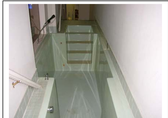
This photo illustrates a corded microphone installed in the baptistery. The risk of electrocution is present for anyone in the baptistery who could contact the microphone. The microphone in this photo should be relocated and suspended from the ceiling or replaced with a cordless microphone.
