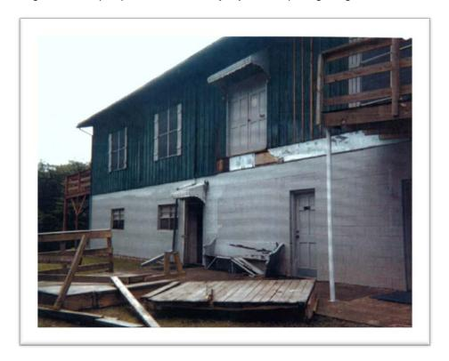
The photo shown here was taken after the accident. Note the complete collapse of the wood deck to the ground and the distance of the fall.
