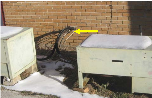
Image above shows an inadequate wiring set up for the central air conditioning units. Electrical is wired directly to the A/C condensing units, without a safety disconnect.
