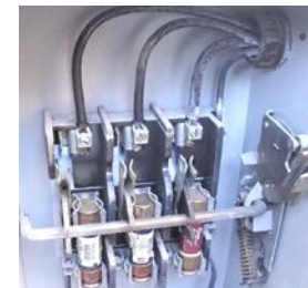
Over current protection—circuit breaker or fuse.
