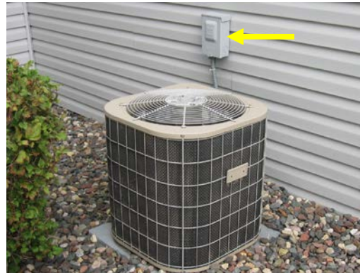
Image above shows the correct installation of an electrical safety disconnect switch.
