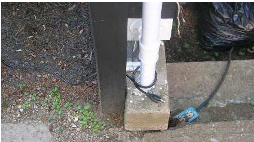
This image shows an outdoor wiring installation that is not a GFCI protected receptacle.
