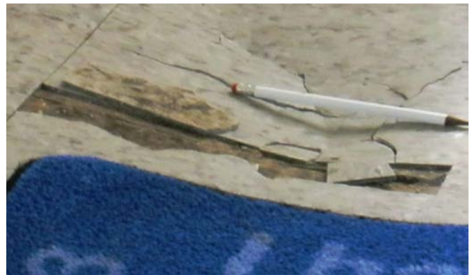
This photo shows an elevated floor that has decayed from inadequate ventilation below the floor surface. Note the collapsing of the floor.
