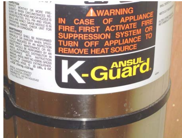
This is an example of a Class K fire extinguisher. Note the warning to only use after suppression system has been activated.
