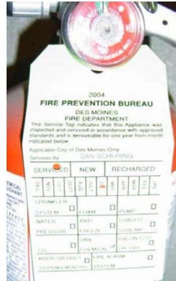
The above photo is an example of a fire extinguisher inspection tag
