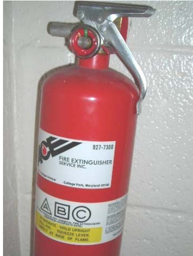
This is an example of a Class ABC multi-purpose rated fire extinguisher.
