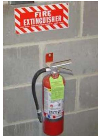
The photo above is an example of a fire extinguisher properly mounted to the wall, easily identified and accessible.
