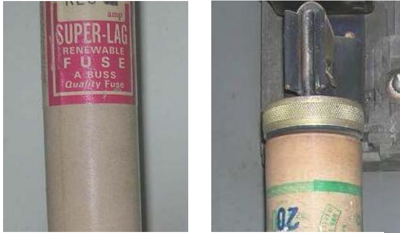
A renewable fuse is a cartridge style fuse that can be identified by labeling (image on left) and/or by the end caps that can be unscrewed (image on right)
