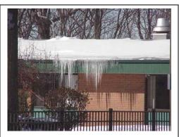
The formation of icicles is a good indicator that there is poor insulation/venting in the attic area. This can lead to water damage.
