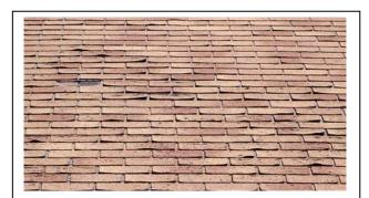
These asphalt shingles are missing, cupping, and blistering. The condition of this roof poses an increased potential of water damage to the interior of the building. Adequate repairs should be made by a qualified roofing contractor.
