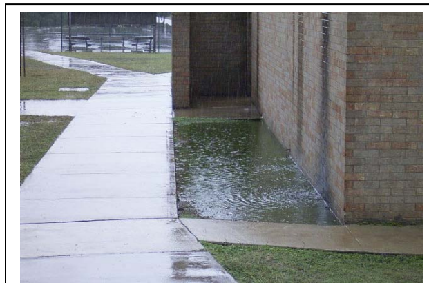
This photo shows inadequate slope and drainage around the building's foundation. Allowing water to settle around the base of the foundation can cause serious water damage to the basement/foundation of the building.
