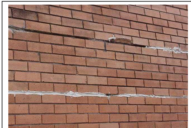
This photo is an example of the wrong way to seal joints in brick. Caulking has been applied to some of the joints. Tuck pointing is needed to repair the mortar joints that have deteriorated by cutting out the old mortar to a uniform depth and placing new mortar in the joints.
