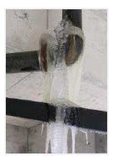
Severe weather conditions: Monitor the temperature where piping could be exposed to freezing. If possible, leave attic access doors open and remove ceiling tiles to keep areas where pipes are located above freezing temperatures.
