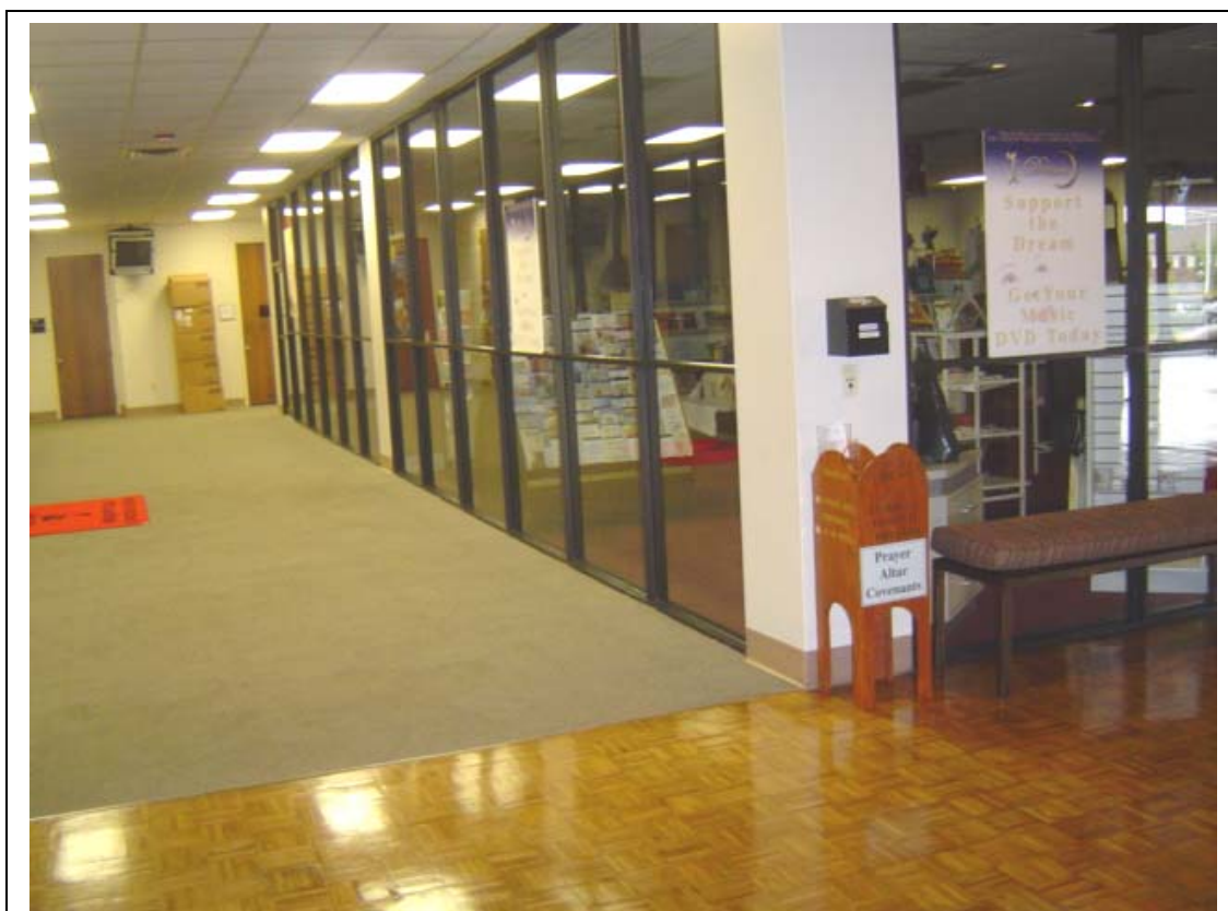
This photo shows a difference in flooring surfaces from carpet to wood tile. Potential slip and fall hazards exist due to the different flooring surfaces installed in a common pathway. Ideally, the surfaces should be consistent. Also note the high degree of smoothness to the hardwood flooring, which also could lead to a slip and fall.
