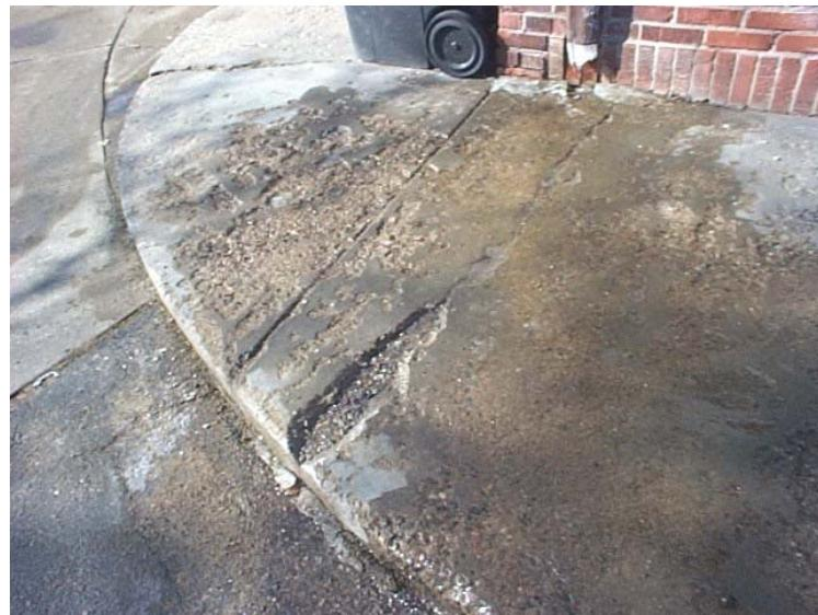
This photo shows the effects of a downspout discharging water onto the sidewalk. This creates an unnecessary wet surface and has badly deteriorated the walking surface. To eliminate the slip and fall potential, route gutters away from any walking surface, and make repairs to the sidewalk surface.
