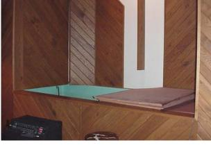
The above baptistery is a good example of providing a carpeted surface around the tank to reduce slips and falls as individuals enter and exit the tank. However, this tank still poses a slip and fall hazard as there are no handrails for the steps leading into the baptistery. The lack of handrails will significantly increase the likelihood of a fall.
