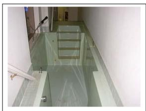
This photo illustrates a corded microphone installed in the baptistery. The risk of electrocution is present for anyone in the baptistery who could contact the microphone. The microphone in this photo should be relocated and suspended from the ceiling or replaced with a cordless microphone.
