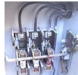
Over current protection—circuit breaker or fuse.
