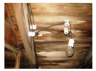
This image shows knob and tube wiring supplying power to a light fixture.
