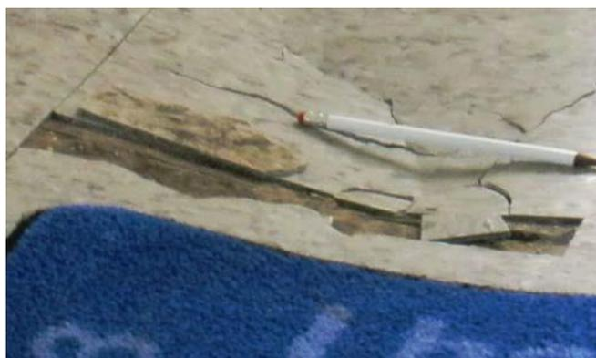
This photo shows an elevated floor that has decayed from inadequate ventilation below the floor surface. Note the collapsing of the floor.
