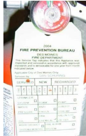
The above photo is an example of a fire extinguisher inspection tag
